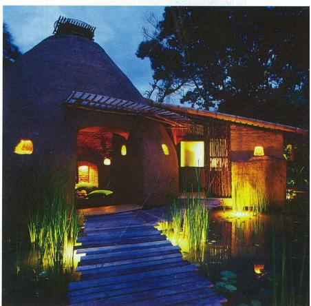
combined with modern techniques. Their low openings on the outside allow refreshing breezes and energy flows to enter the buildings, while the openings at the top of each provide natural ventilation. The project achieved a holistic integration of green design, aesthetics, involvement of the local community and knowledge transfer from one geographical region to another,
